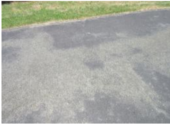
Uneven wearing of seal coat.
