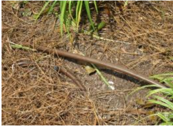
Exposed irrigation lines.
