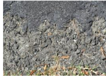
Seal coat not applied to edges.
