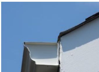
Inadequate overhang of shingles.
