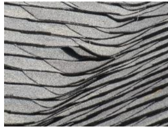
Shingles not laying flat properly.
