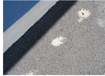
Patching of holes in asphalt.
