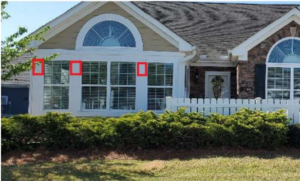
CANTERBURY (Original Design) Buildings 2, 3, 4, 5, 6
