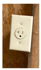
It appears someone installed a higher amp/volt outlet on the wasll of the pump room. it appears this was probably for a space heater at some point prior to the pool being covered and winterized.
