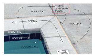
Having a <u>3/4 caulked expansion joint</u> between your pool deck and your pool coping prevents cracking in both, and protects the waterline tile from movement in the deck, Pouring the deck and the coping all together is a costly shortcut many developers take.
