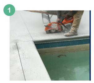
Saw cut around full perimeter of the pool creating separation between the coping and the pool deck.
