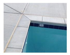
As you can see from images, the work of replacing the coping and waterline tile at your pool, must be done with the pool empty and is best completed prior to resurfacing your pool to protect the new surface we will be installing. We can resurface the pool without doing the coping and waterline tile work, but for best results, all of these scopes should be done together.
