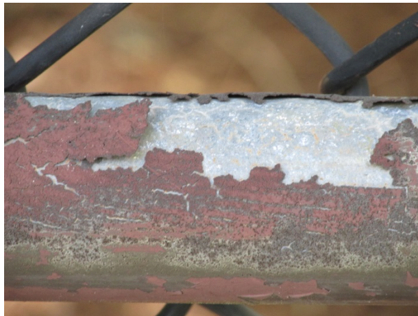
Fence – Note rust and chipped paint
