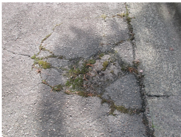
Cracks and settlement of pavement
