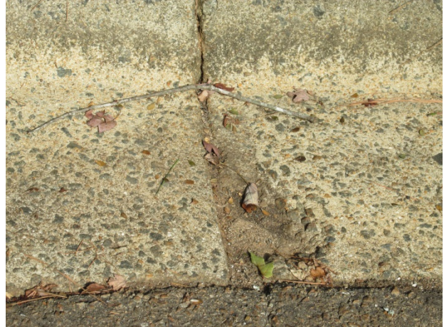
Concrete gutter – Note spalled concrete
