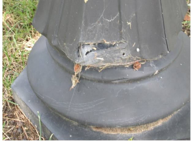
Base of pole – Note damage
