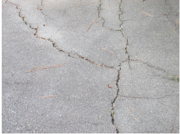
Cracks in pavement
