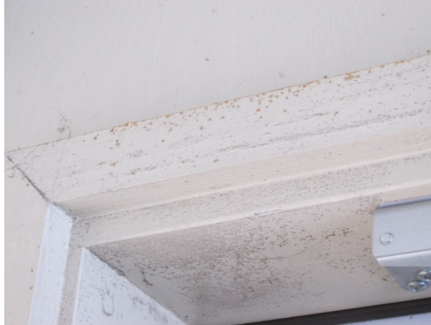
Paint finish – Note weathered paint
