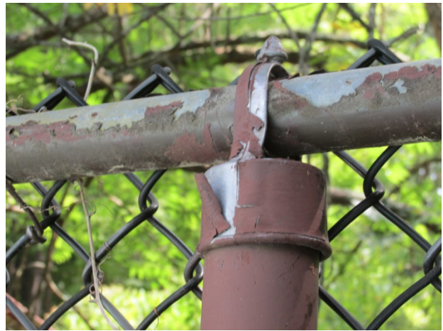
Fence post – Note rust and chipped paint
