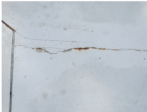
Concrete deck – Note crack
