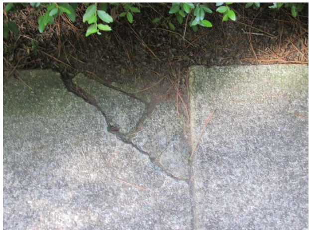
Sidewalk – Note cracks and settlement
