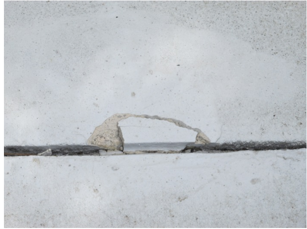
Concrete deck – Note chipped concrete
