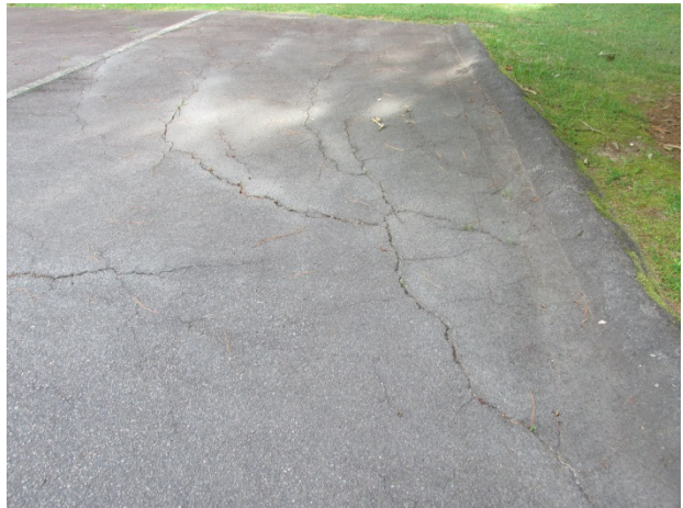
Settlement of pavement – Note slippage
