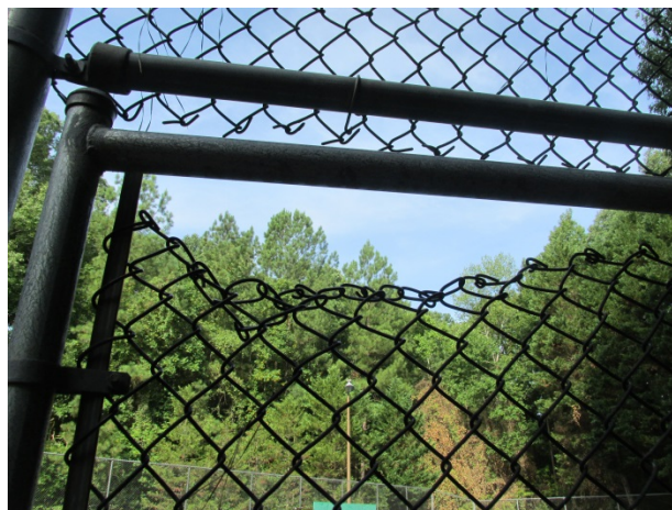
Fence – Note warped webbing
