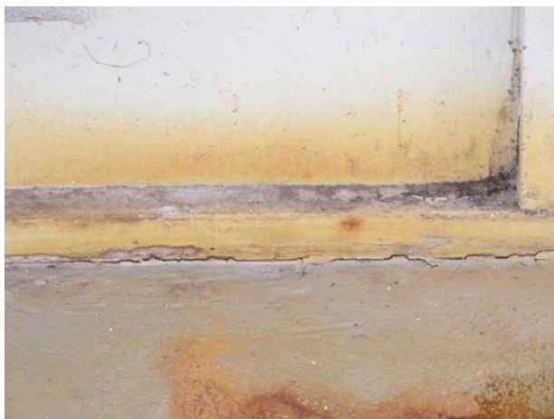
Siding – Note damage under wall mounted drinking fountains
