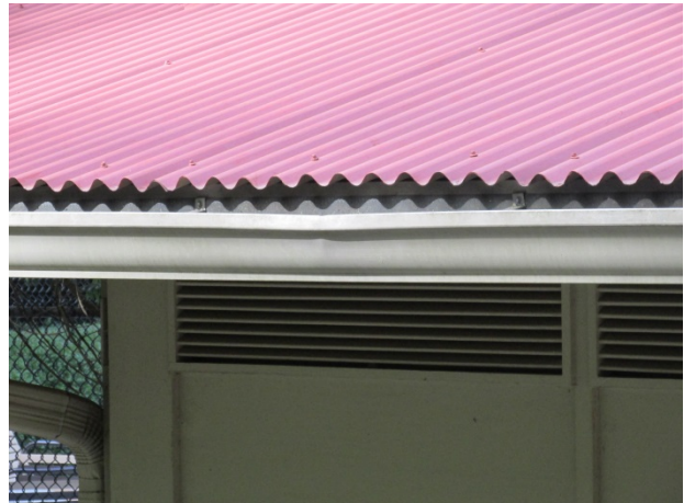
Metal roof and gutter – Note dent in gutter
