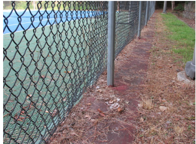
Fence – Note warped webbing
