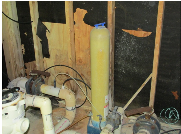
Automatic chlorinator
