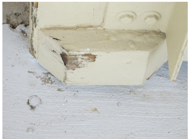
Paint finish – Note chipped paint
