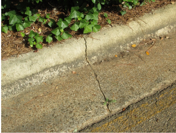
Concrete curb and gutter – Note crack
