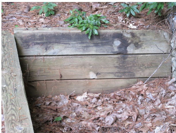
Wood retaining wall – Note water stains
