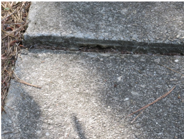
Sidewalk – Note trip hazard
