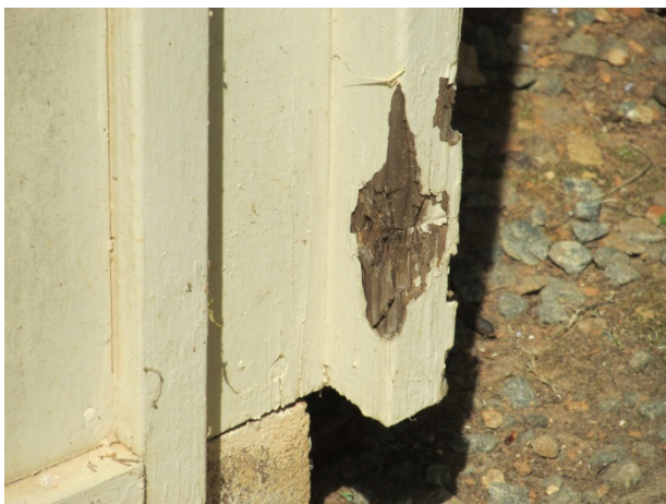
Damage to siding on the maintenance shed
