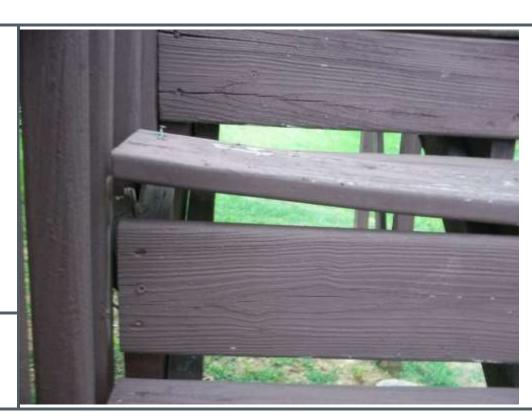
Example of deterioration in deck boards.
