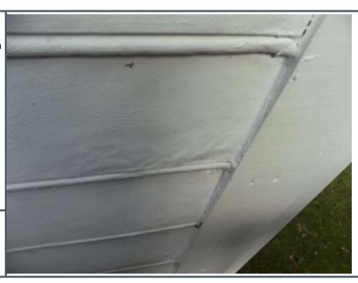
View of caulking at butt joint and minor swelling in lap siding at butt joint.
