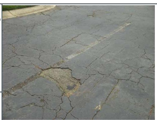
Example of fatigue cracking in asphalt paving.
