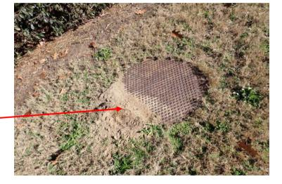
Picture: Treatment Area Tasks: 1 Remove sand/sediment from area 2 3 Remove all sediment from underground detention system, as specified by O&M Manual
