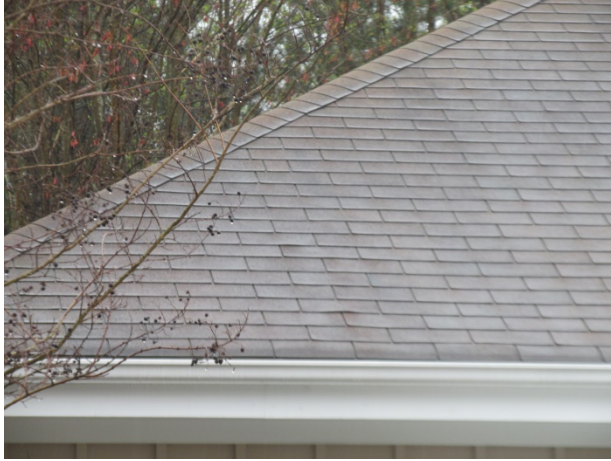
Shingle lift evident
