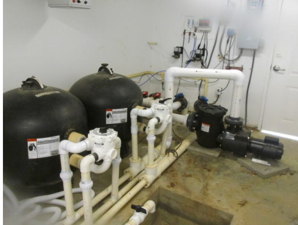
Pool pumps and filters
