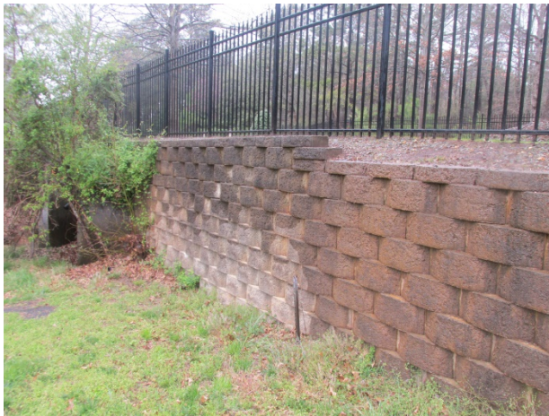
Masonry retaining wall
