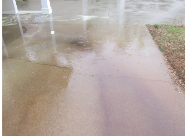
Cracks evident
