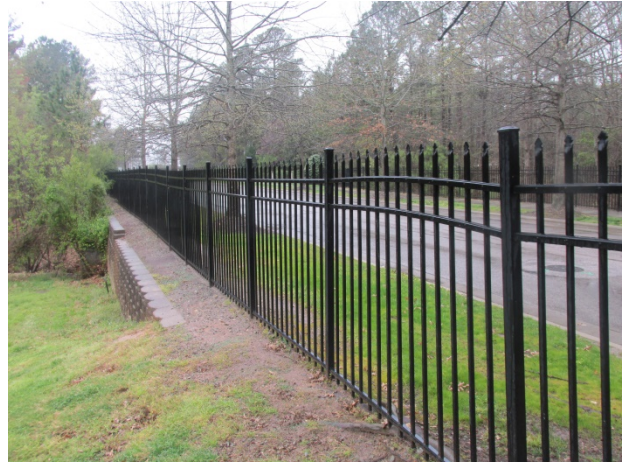
Aluminum fence at masonry retaining wall
