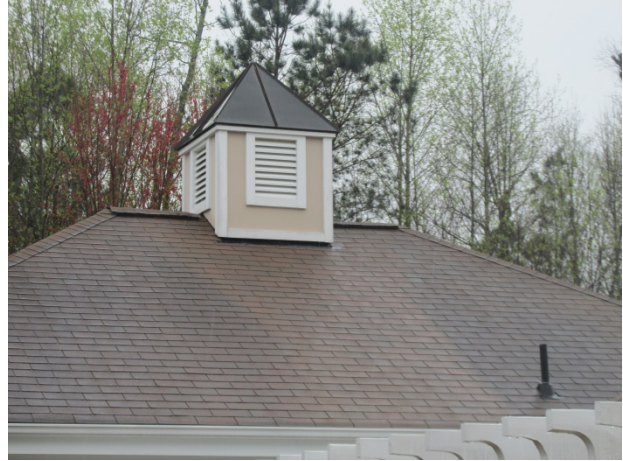
Asphalt shingle roof overview and metal cupola
