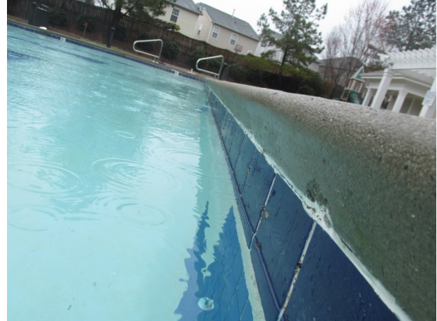
Plaster and tile at the pool perimeter
