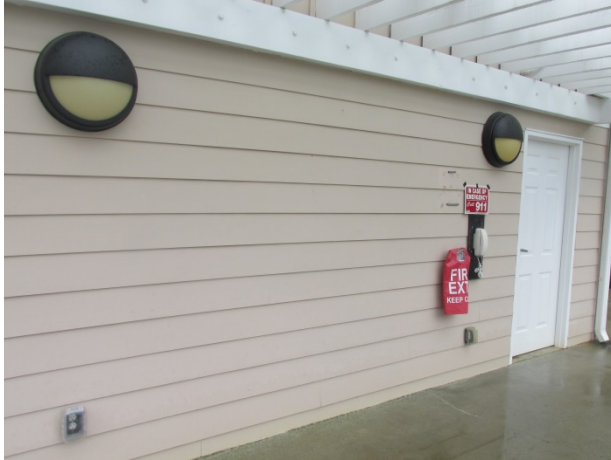
Fiber cement siding
