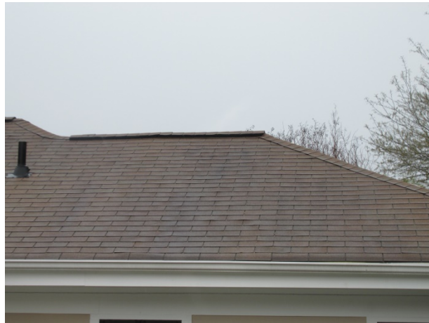
Shingle lift evident
