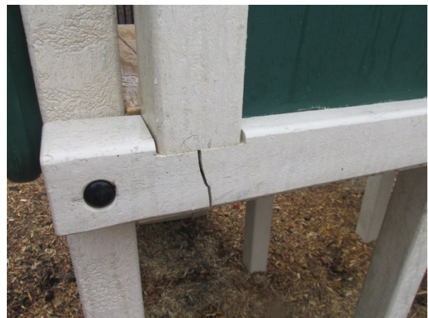
Cracks evident
