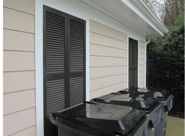
Fiber cement siding
