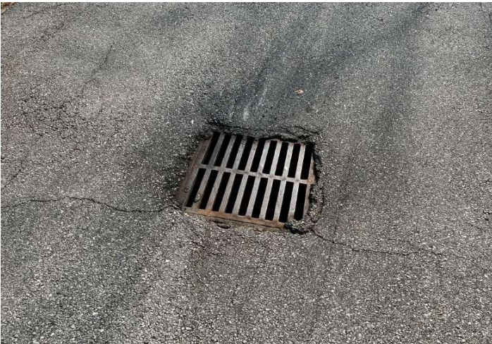
Catch basin at recently overlaid pavement
