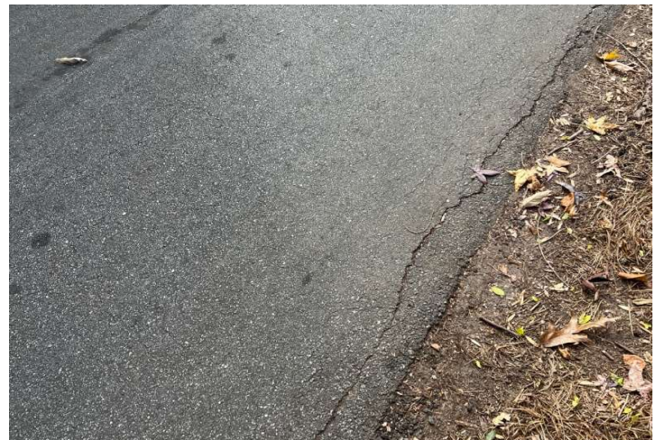
Small crack at edge
