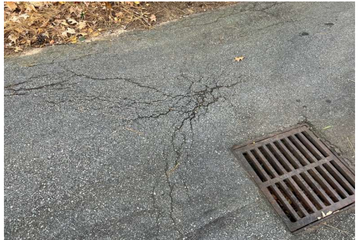
Small deterioration adjacent to catch basin
