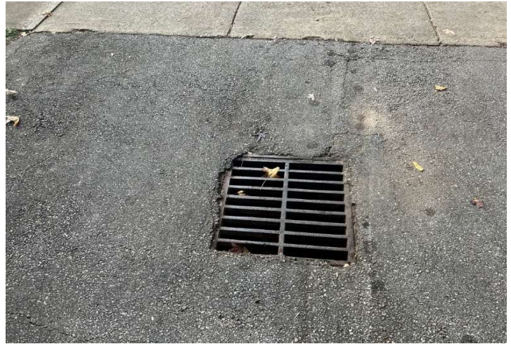
Typical inlet at end of alley
