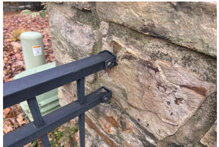
Connection at masonry column
