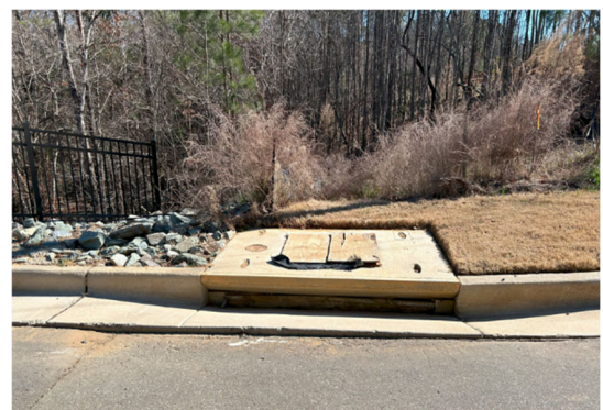
Figure 13: High Woods Ridge Road Curb Inlets
