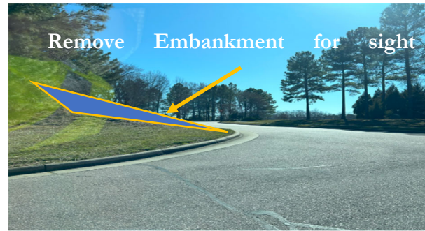
Figure 8: Obscured Sight Distance Rolling Meadows at Covered Bridge Trail
